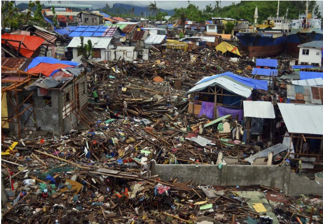
City of Tacloban in the Philippines, damage done by the Typhoon Haiyan (source: Britannica)
