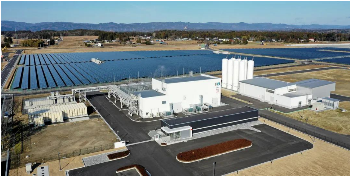
The world's largest green hydrogen plant, Fukushima, Japan.
